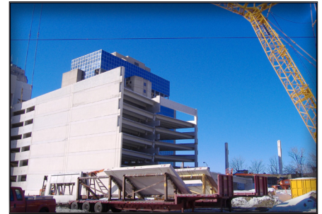
750 Court Street Parking Garage City of Reading
